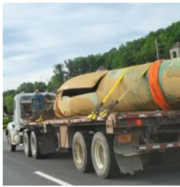
Safety, oversight questions linger after Mountain Valley Pipeline rupture
