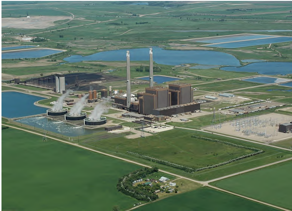
Coal Creek Station
