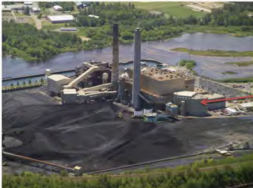
Presque Isle Power Plant
