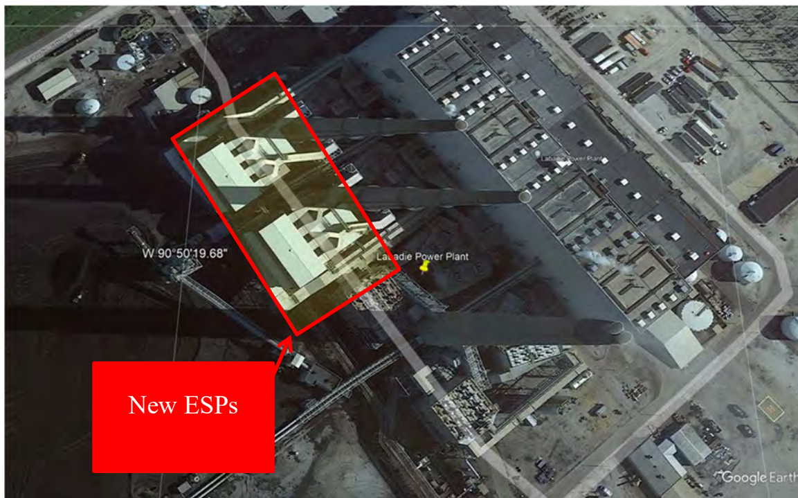
Figure 13. New ESPs at Labadie units 1 & 2 and adjacent units 3 & 4 with older ESPs. 89
