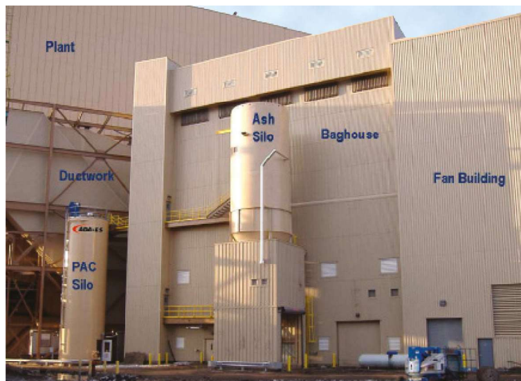
TOXECON™ System Installed at PIPP
