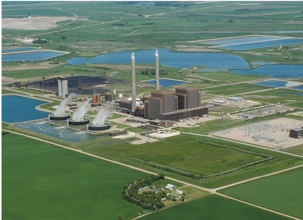
Coal Creek Station
